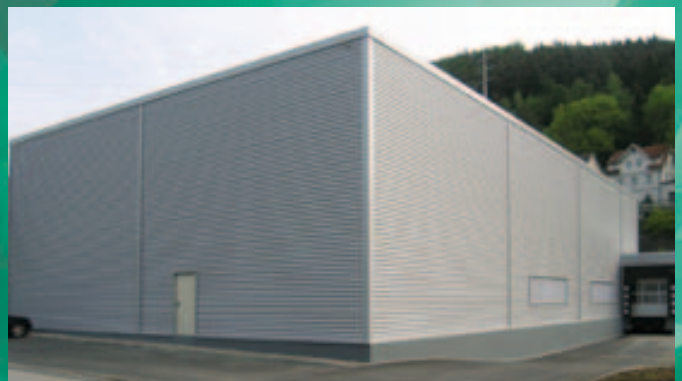
Eickemeyer Logistic Centre in Tuttlingen, Germany
